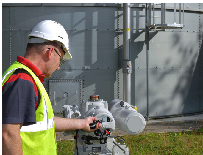
Figure 1. An engineer commissions the actuator using its integrated display and menu system.
