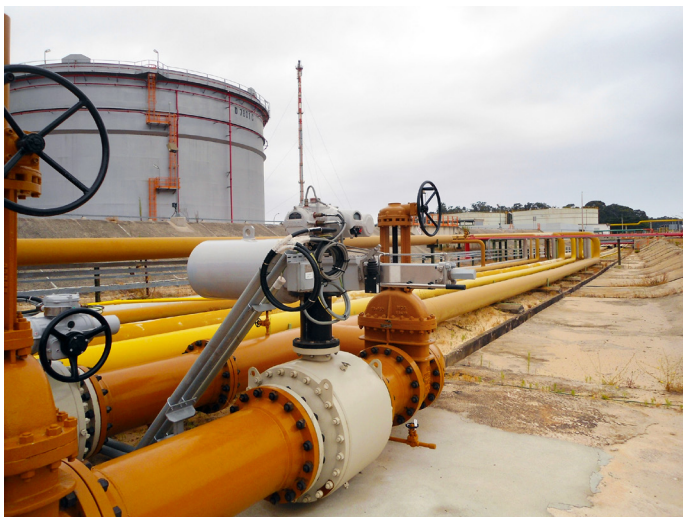
Figure 2. Self-contained electro-hydraulic actuators for safety-critical and fail-safe applications.
