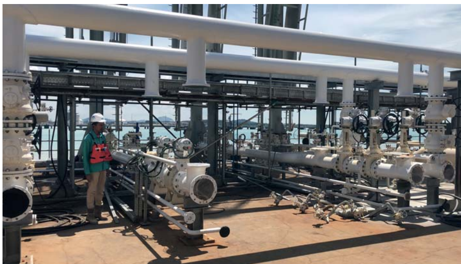
Some of the IQ3 actuators at the terminal during installation.
